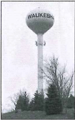
A Waukesha water tower on Meadowbrook Road.
