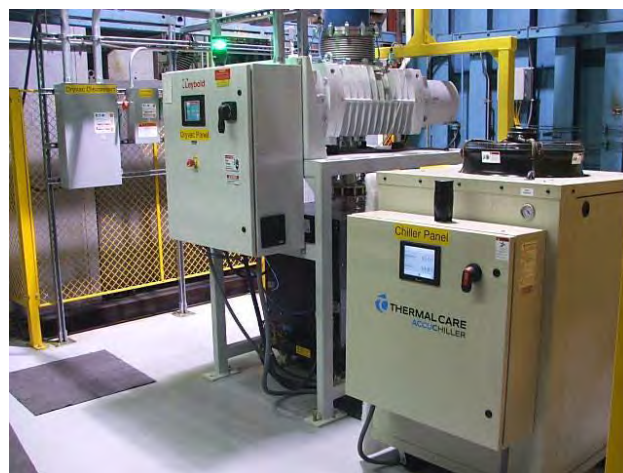
Eaton's 3 rd Recirculating Water Chiller
