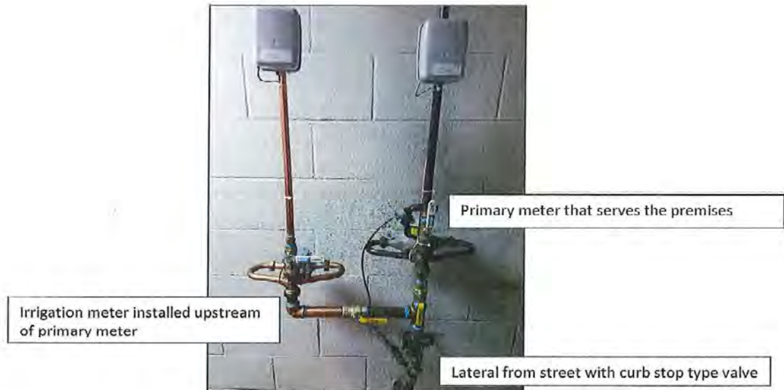
Installation of a 5/8 inch irrigation meter
