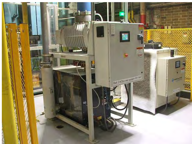
Eaton's 2 nd Recirculating Water Chiller
