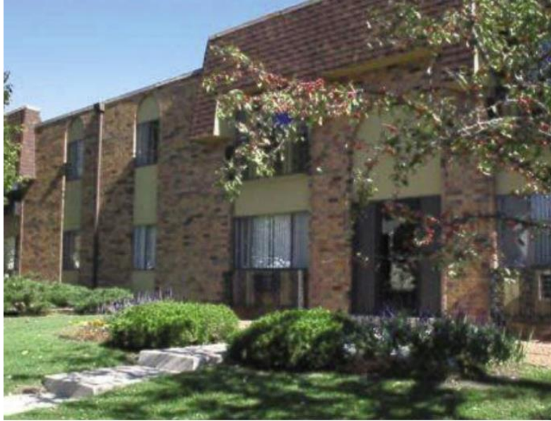
The Equity Group's First Complex – changed out 20 toilets dating from 1968-1991.
