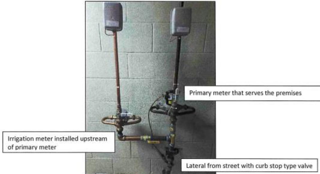
Installation of a 5/8 inch irrigation meter
