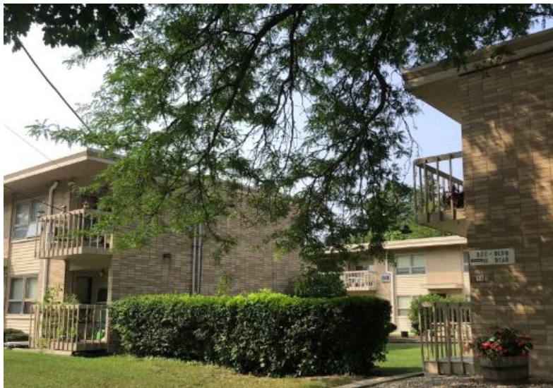
The Equity Group's Second Complex – changed out 37 toilets dating from 1965-1973. The majority of the toilets were from the mid-1960's.
