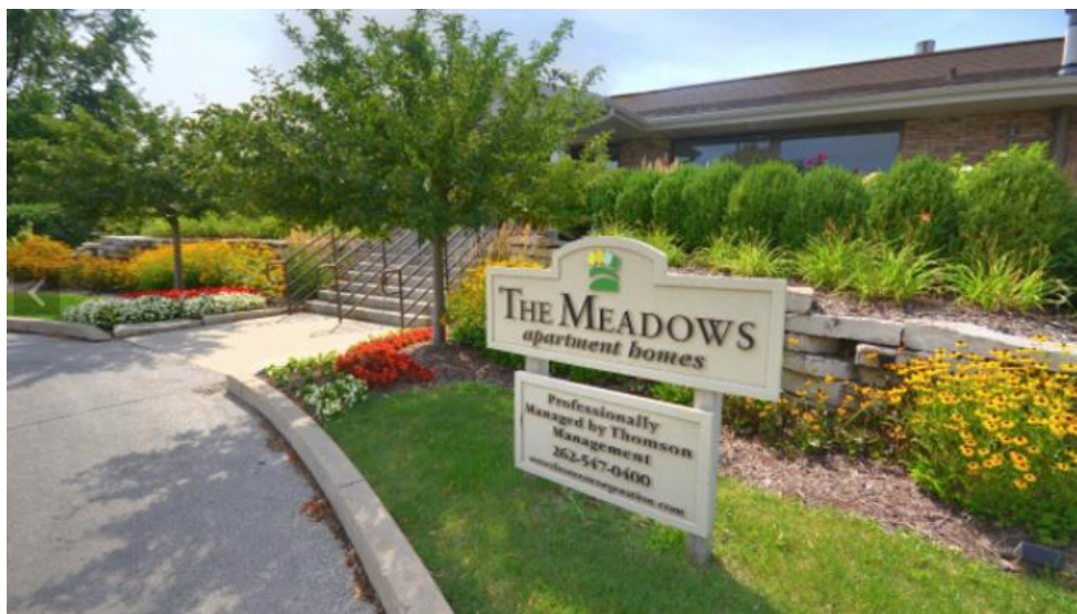
The Meadows Apartments changed out 83 toilets – most of the toilets dated back to 1972, but a few were dated 1991.
