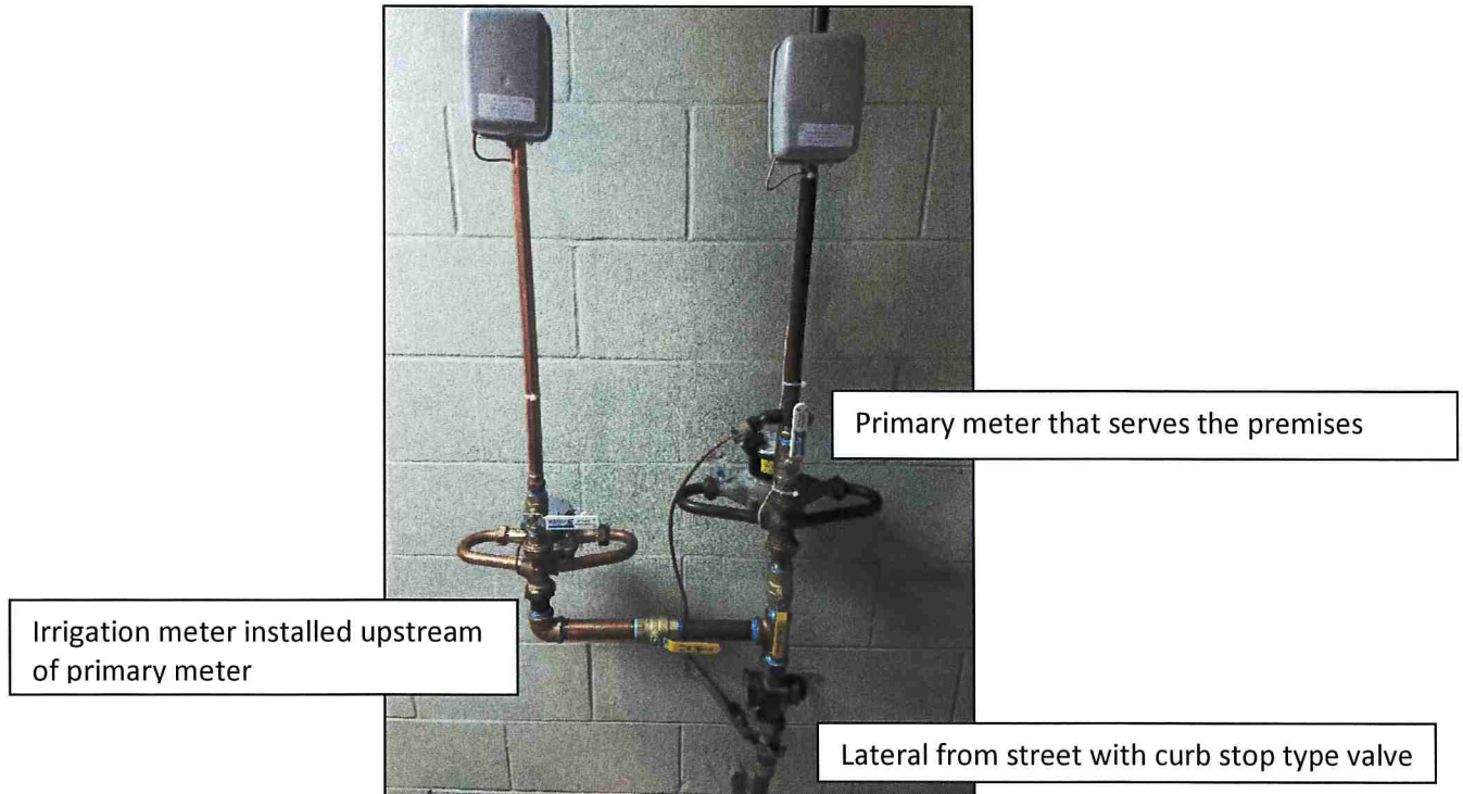
Installation of a 5/8 inch irrigation meter
