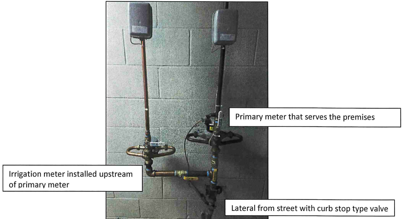
Installation of a 5/8 inch irrigation meter
